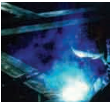
Figure 5 MMA welding can produce large amounts of particulate fume
